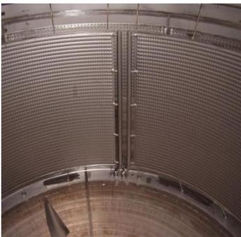
Figure 3: Additional heat exchange plates (GEA Brewery Systems)
