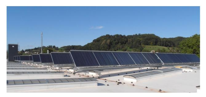
Figure 13: Field of 80 high performance evacuated tube collectors with CPC reflectors on the roof of Zehnder in Gränichen, Switzerland, with a gross area of 394 m<sup>2</sup> (Source: Ritter XL Solar)
